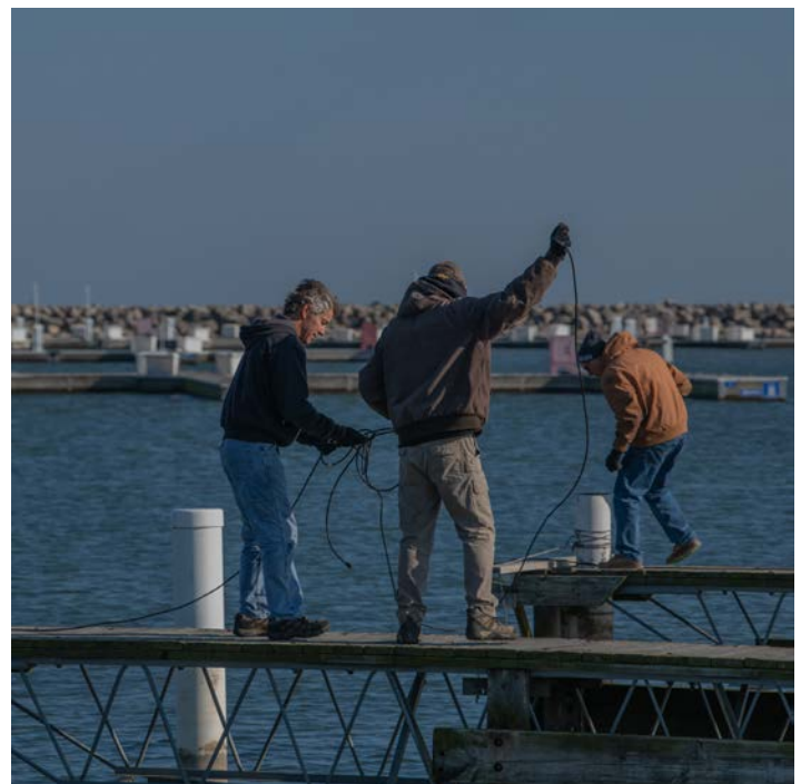
Below: Cory Vertz and Jeff Weis hooking up an agitator on the end of one of the piers
