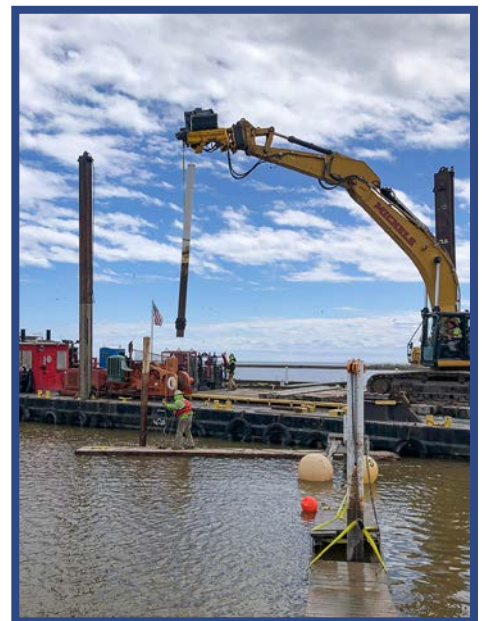
Above and Left and Right: The Michels crew works on raising up the damaged pier as well as relocating and reseating the the remaining pilings. Photos: Jason Diener
